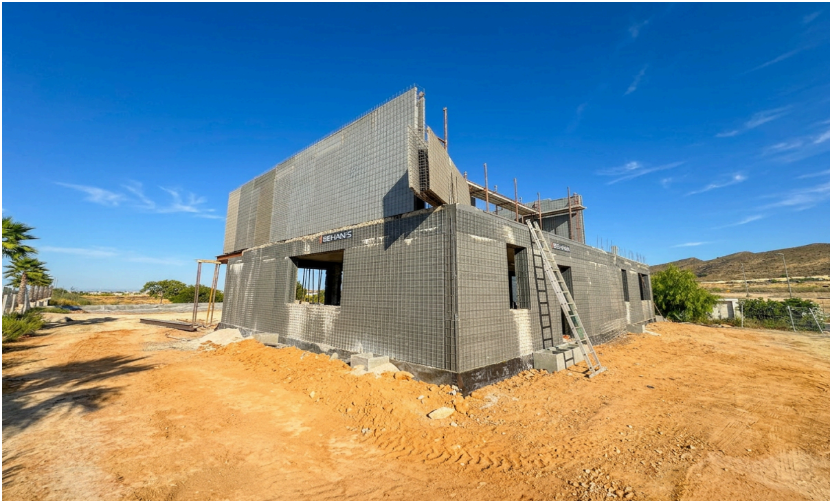
SISMO construction at Altaona — precision engineering built into every wall.
