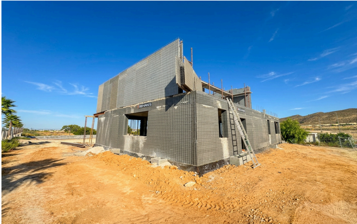
SISMO structural system in progress — precision engineering and superior insulation built in from the ground up
